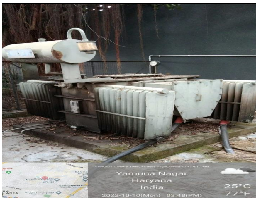
Figure 2.1:- 400 kVA Transformer
